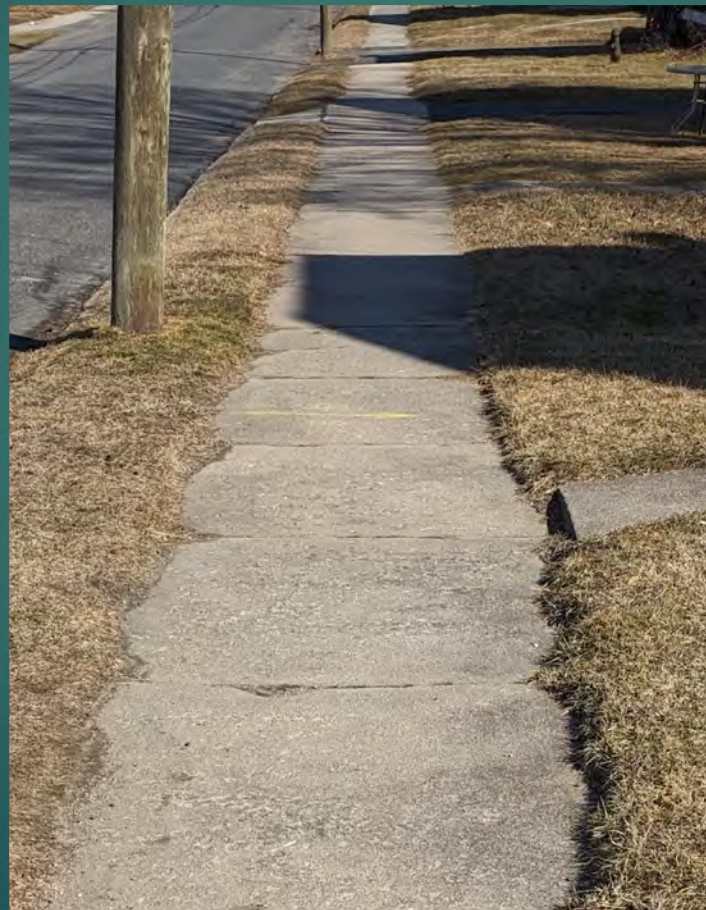
An 84-year-old cement concrete sidewalk on Flansburg Ave, Dalton, MA installed in 1940.
