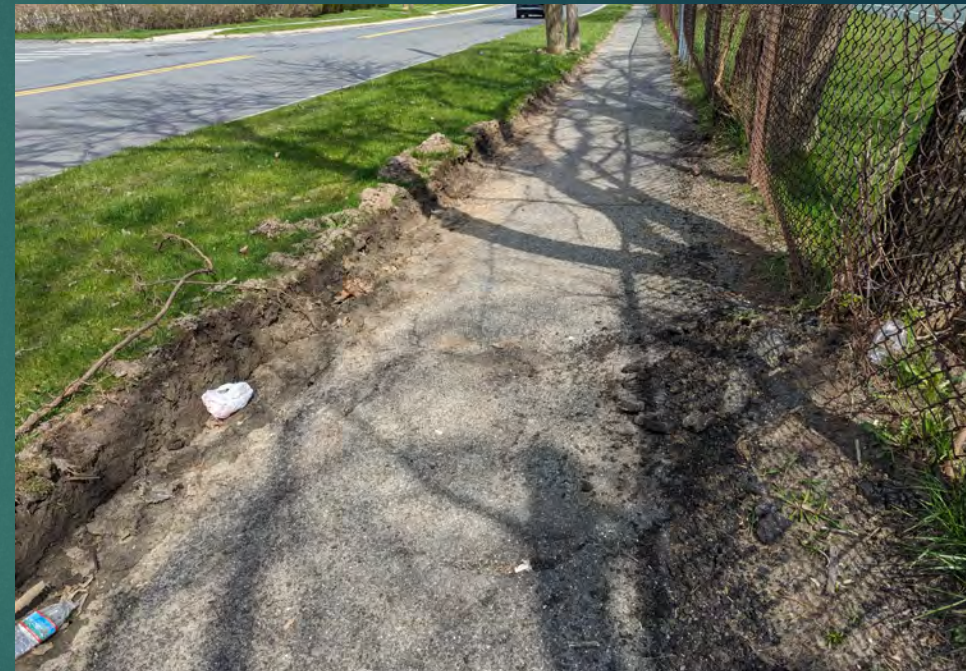
Asphalt sidewalk on Springside Ave, Pittsfield, MA.
